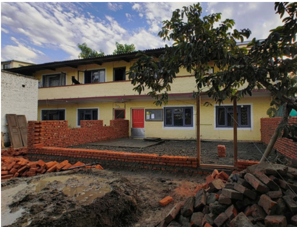
Construction as traditional mud structure
